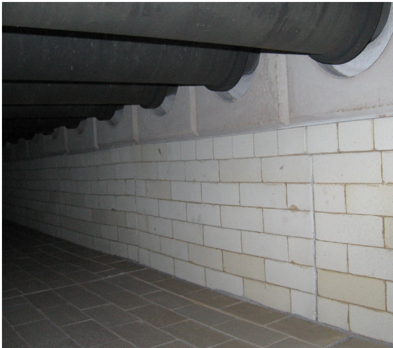
Roller hearth furnace 1050 °C with SILCAREF
